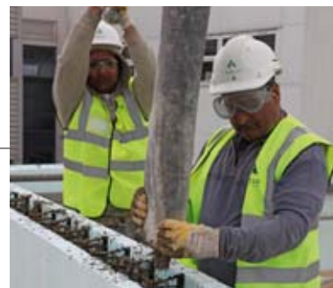
Above: Following pouring, concrete is 'consolidated' using a poker vibrator
