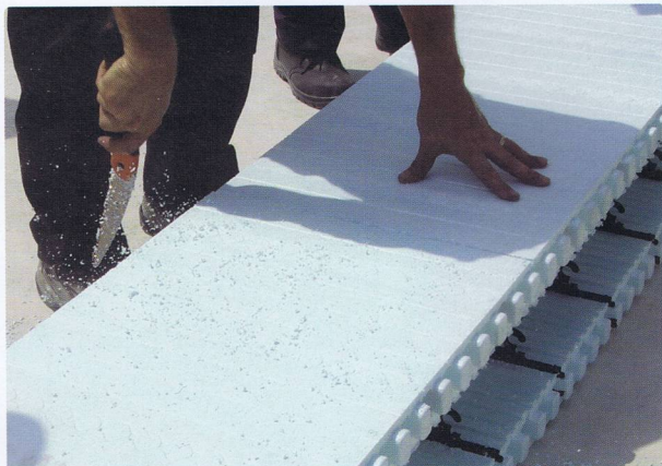
The EPS block can be simply cut to ease installation.
